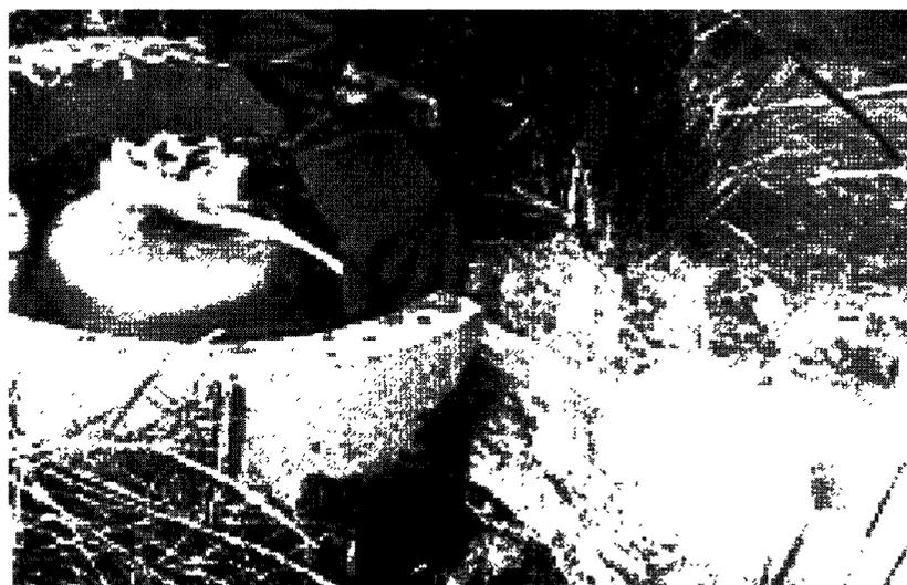
Fig.2 Application of WDG with a mesh bag to a water inlet
